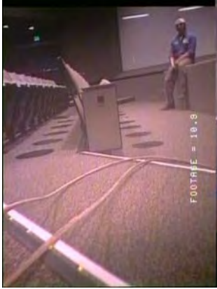
Figure #8 Gallery piping side view
