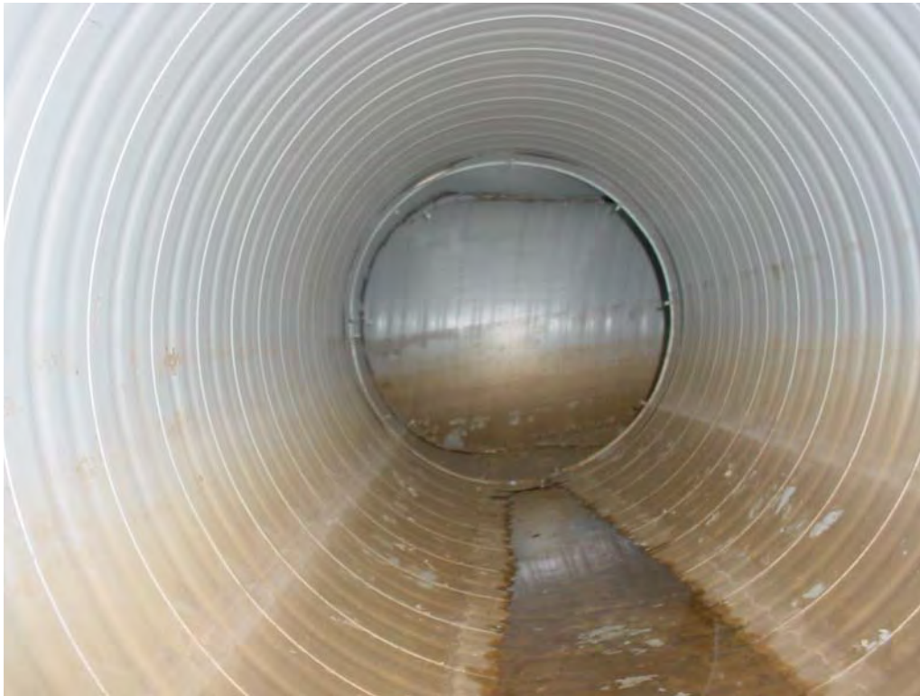
Figure #6 Pre Video of plenum junction
