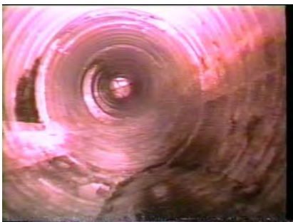
Figure #10 Internal mildew manifestation
