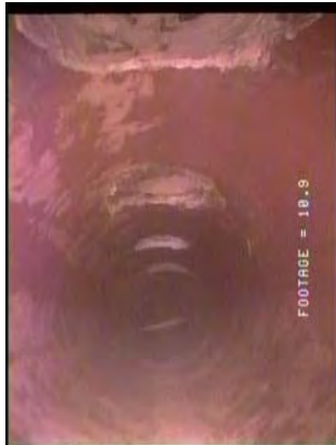
Figure #2 Post Video of Air Plenum cross run
