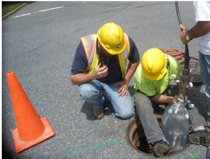
Figure 3. Light Train inserted into a 30-in. Trunk Sewer on Division Street
