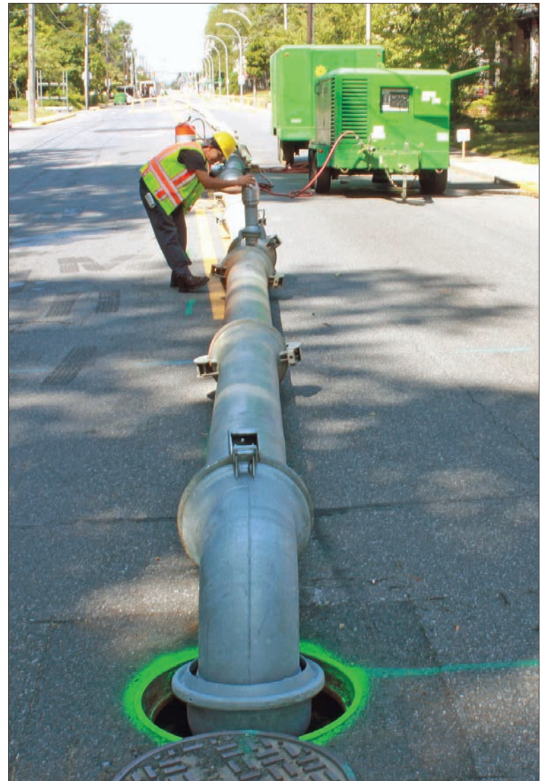
At the end of the mile-long bypass system, a crew member checks the pressure and releases a small amount of air so that the bypass system flows with ease.
