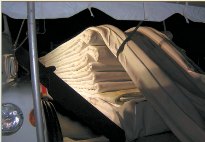
The over the hole inversion technique is used when the tub and resin weigh too much to factory impregnate and haul to the site. Instead, a makeshift plant is assembled over the pit, or hole.
