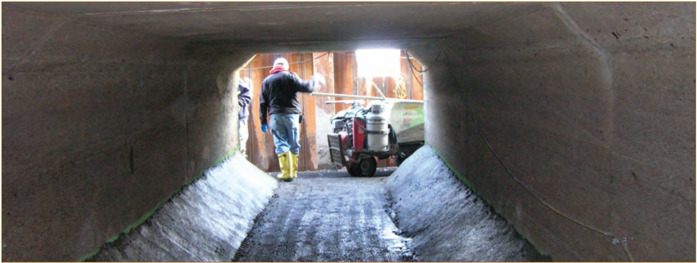
The Joe Campau B 10 Outfall installation that rehabilitated 3,600 lf of a rectangular box culvert in Detroit pushed the boundaries of pipe rehabilitation.
