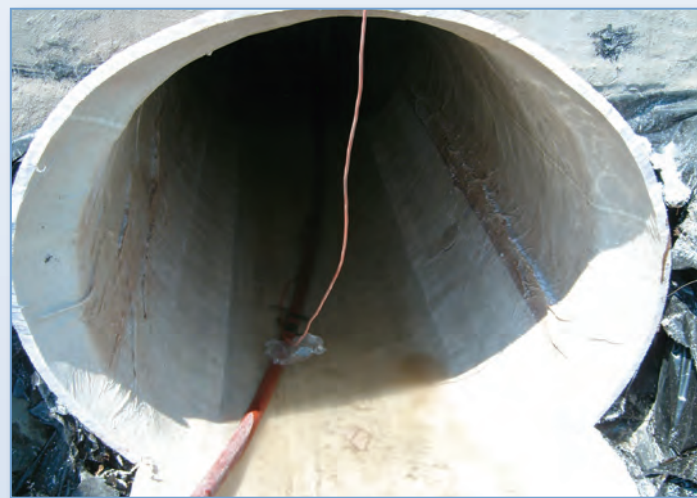
Finished outfall product at the headwall
