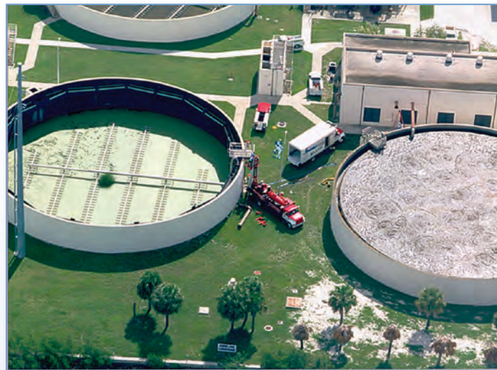
Clarifier pressure pipe rehabilitation at WWTP
