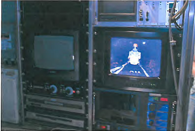
Figure 3. Corp stops are plugged prior to lining
