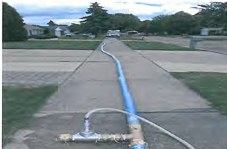
Figure 2. Potable water bypass piping maintaining service to houses
