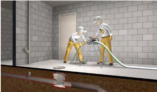
Figure 2: Liner calibration using calibration roller
