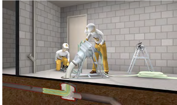
Figure 3: Inversion using the RS LinerGun®
