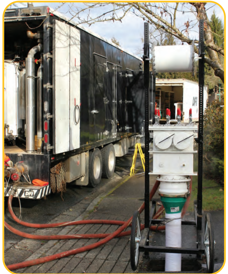
Figure 3: Air inversion of liner
